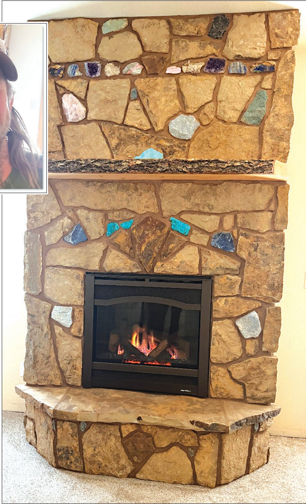
Frazier Family Fireplace-Mike Mackey Stone Masonry
