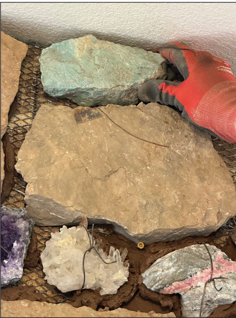
Process of Attaching Stones Before Final Mortar
